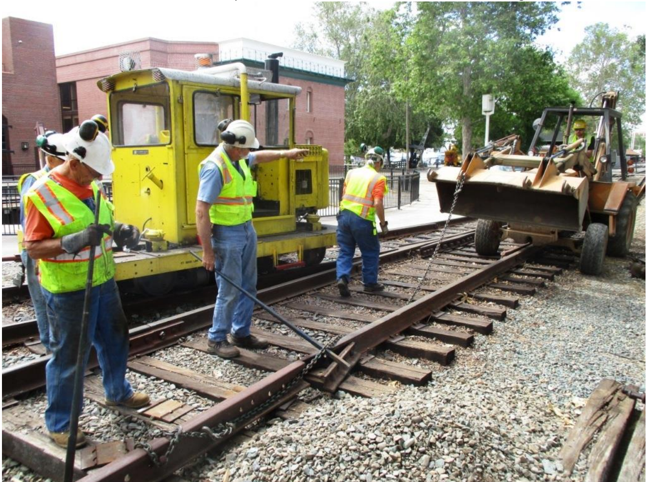
Alan guides the chain as Chris on the back-hoe slides the rail into position right between the spread joint-bars
