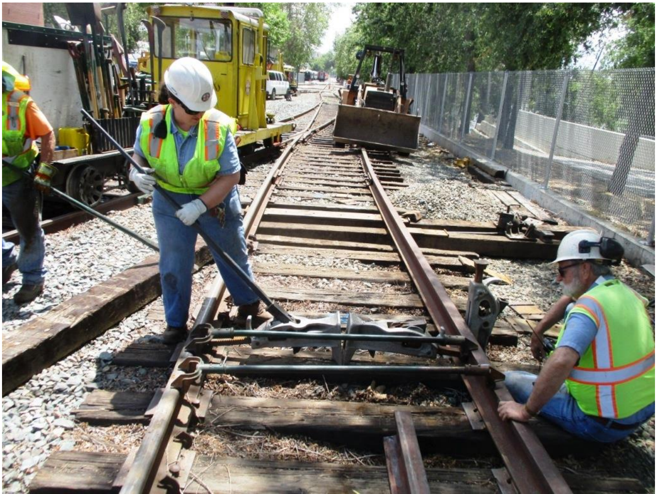
Alan checks the measurements as Heather uses track-jacks to spread the rails into the correct gauge
