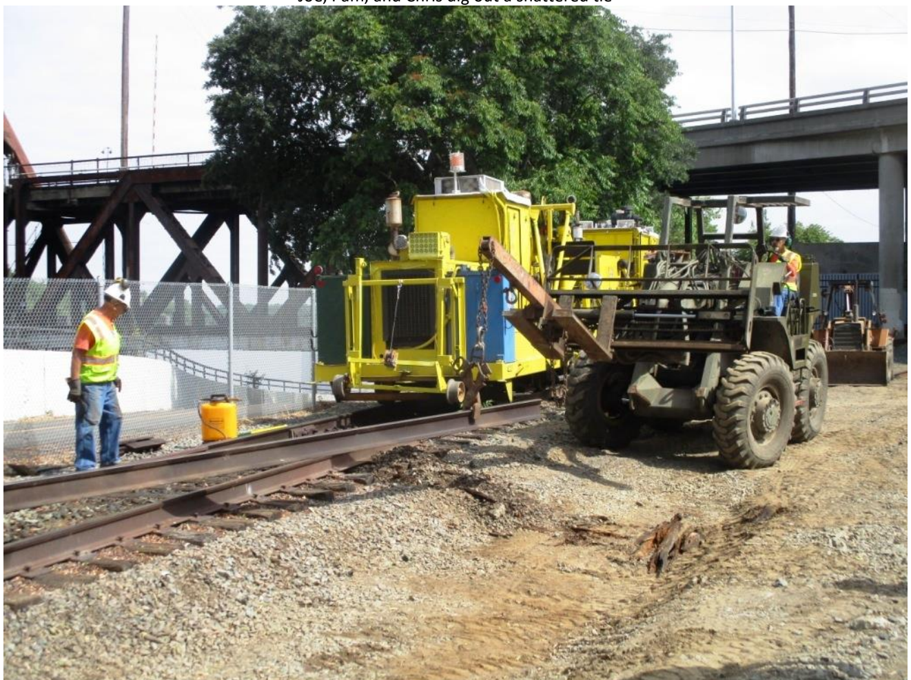
Ed on GM2 removes the cut-out stick of 113-pound rail
