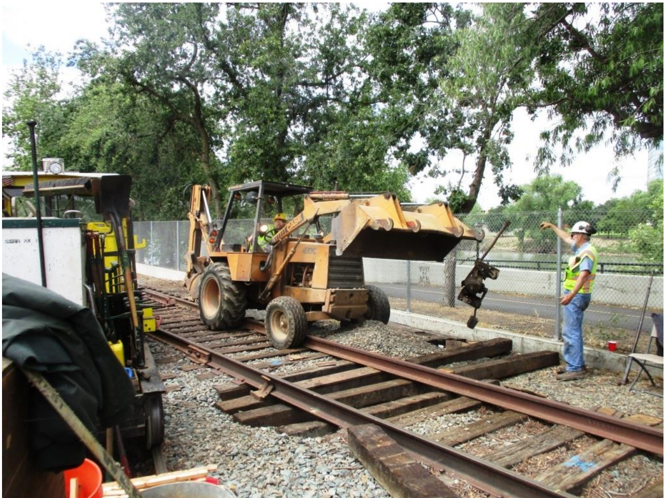
Alan guides Chris on the back-hoe as the ground-throw switch machine is placed on the head-block ties
