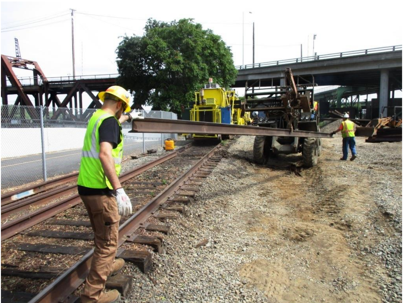
Chris and Clem guide the removal of the old stick 112-pound rail
