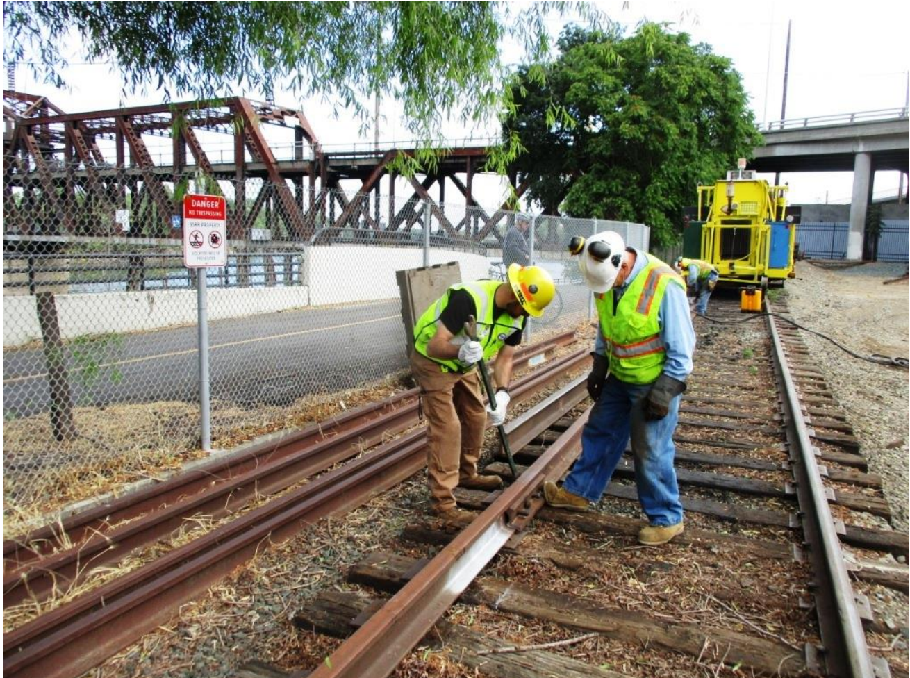
Chris and Clem take apart the north joint of the defective rail
