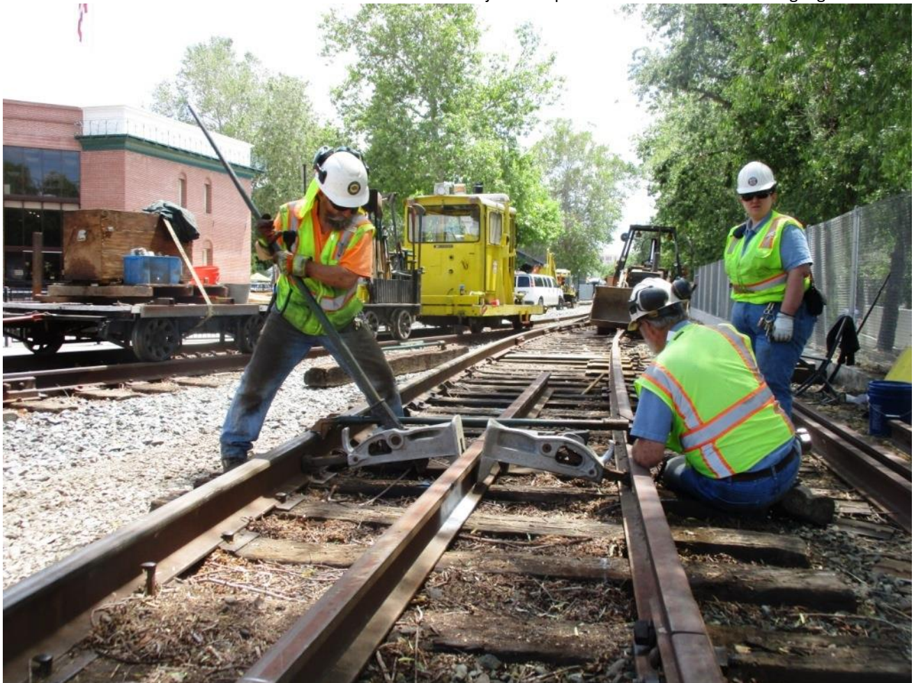
Joe now spreads the rails with track-jacks pressing up against closure rail
