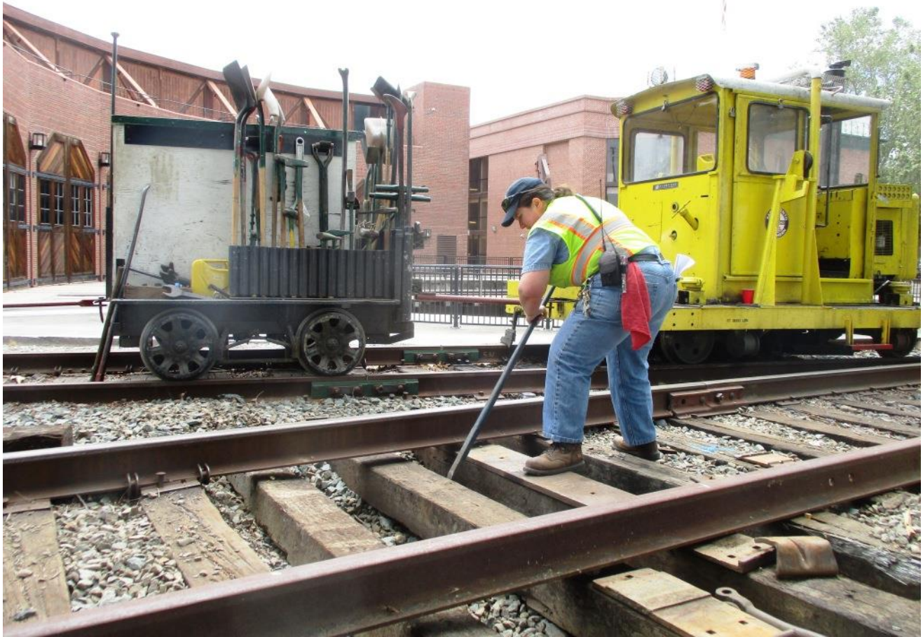
Heather shimmies the head-block ties to the correct distance from each other
