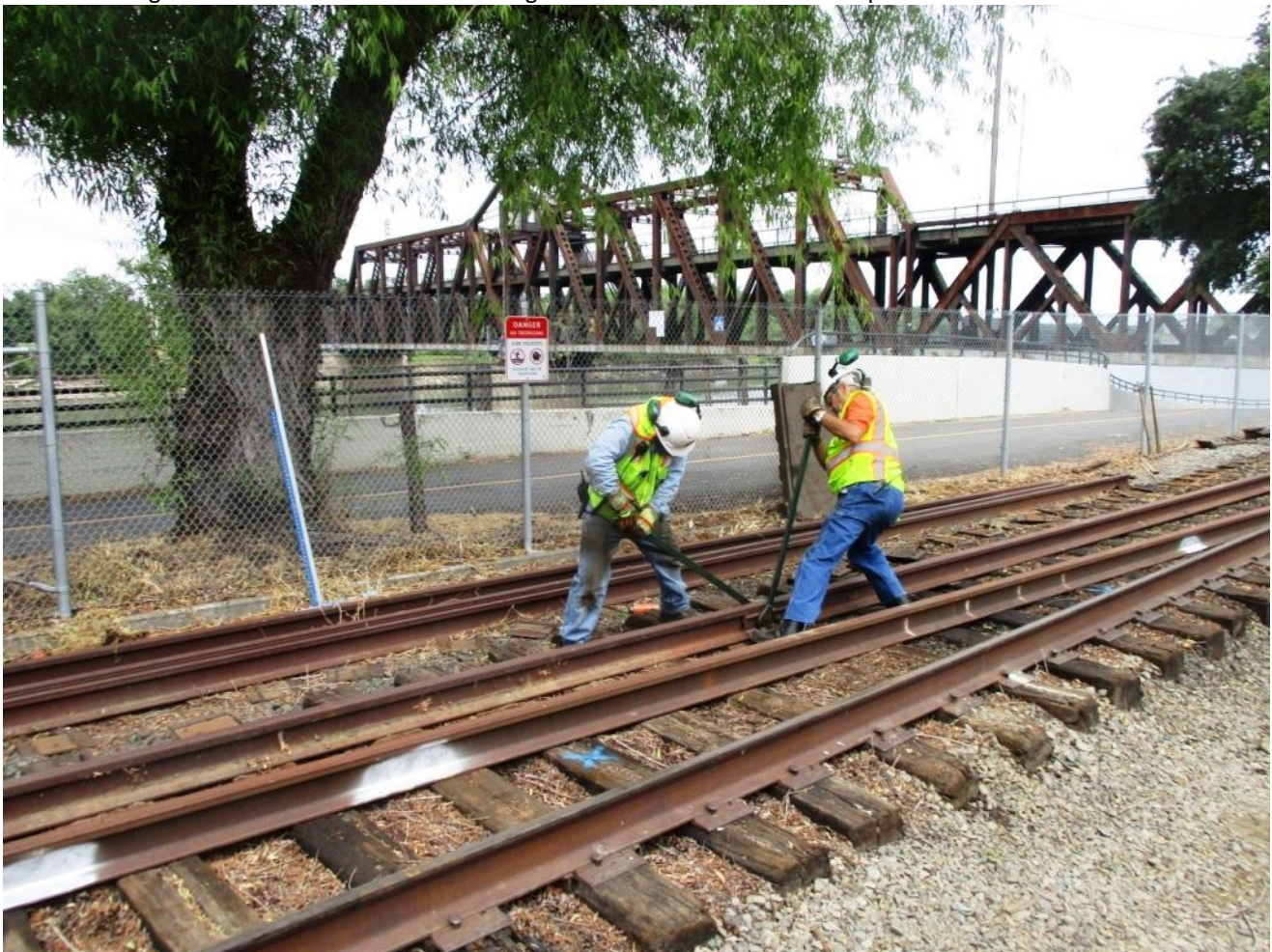
Joe and Ed tighten the bolts at the north joint
