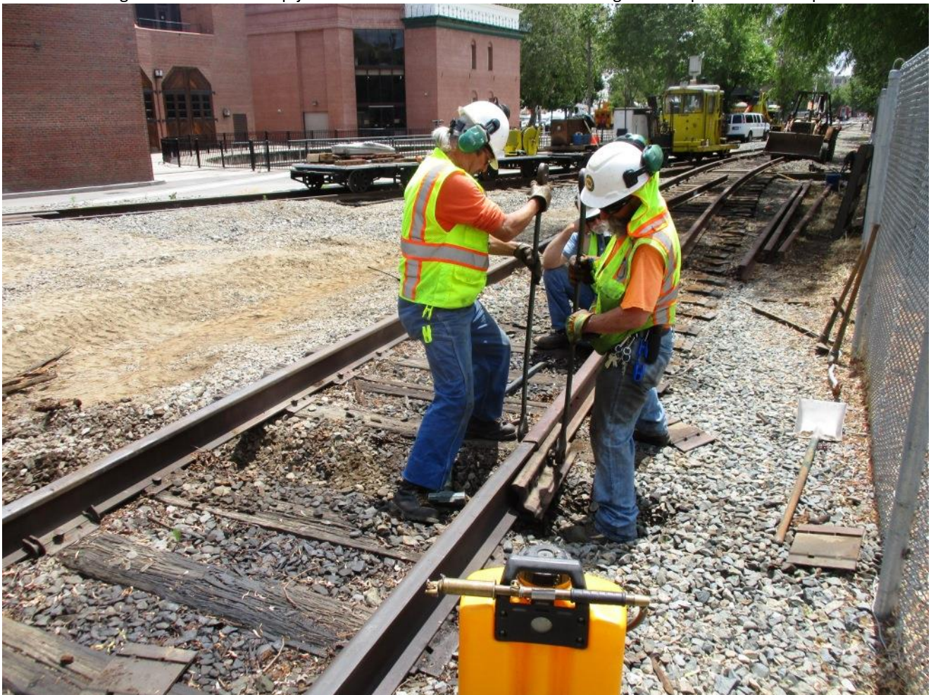
Ed and Joe tighten the bolts on the comp-joint
