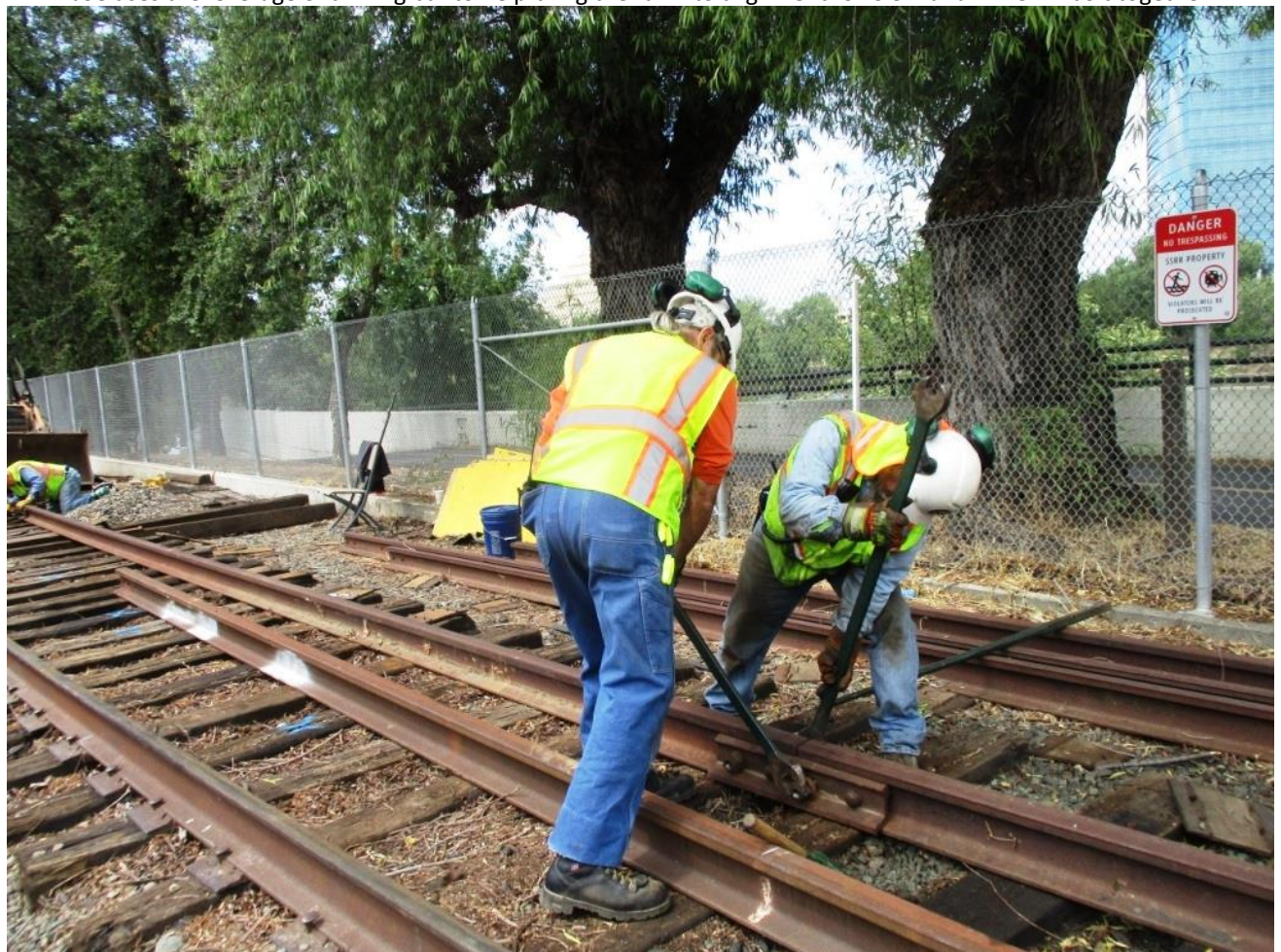
Ed and Joe tighten the bolts
