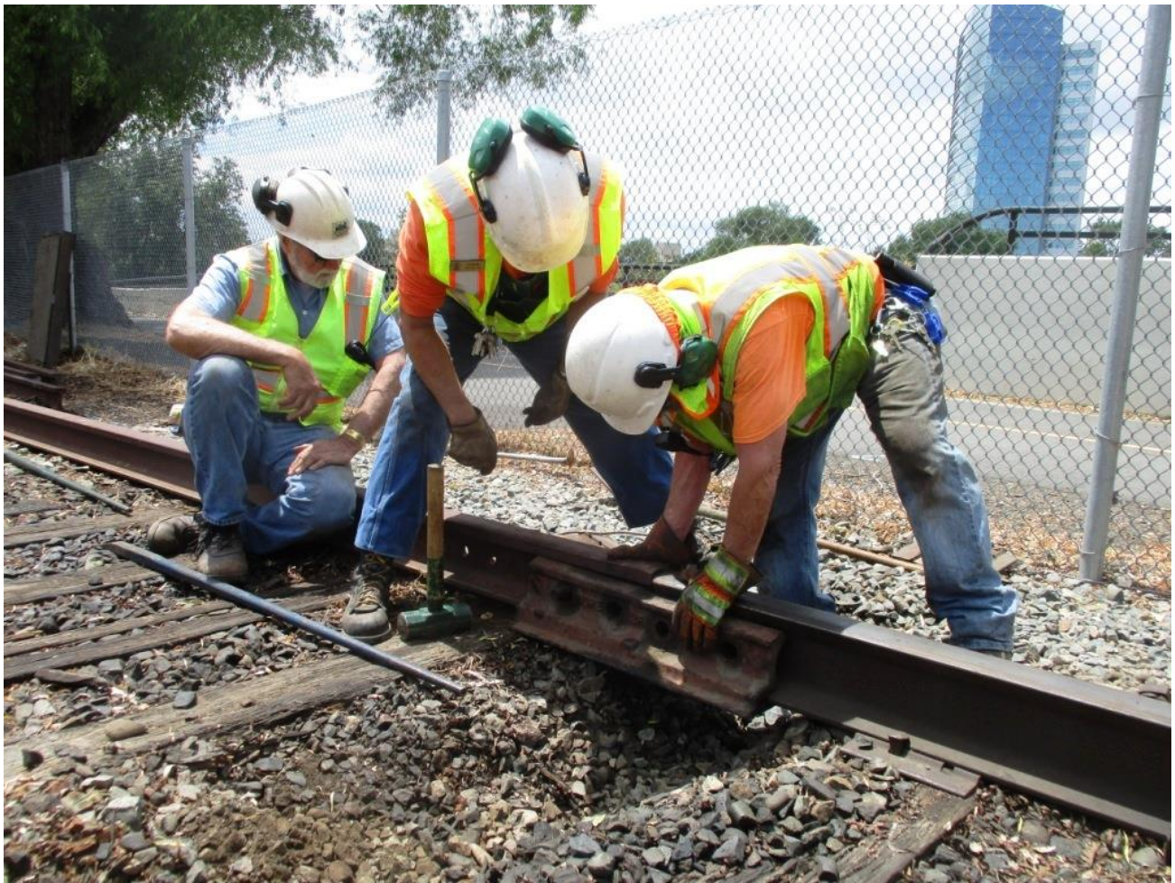
Ed and Joe get the armored comp-joint bars attached to the track connecting the 110-pound and 113-pound rails
