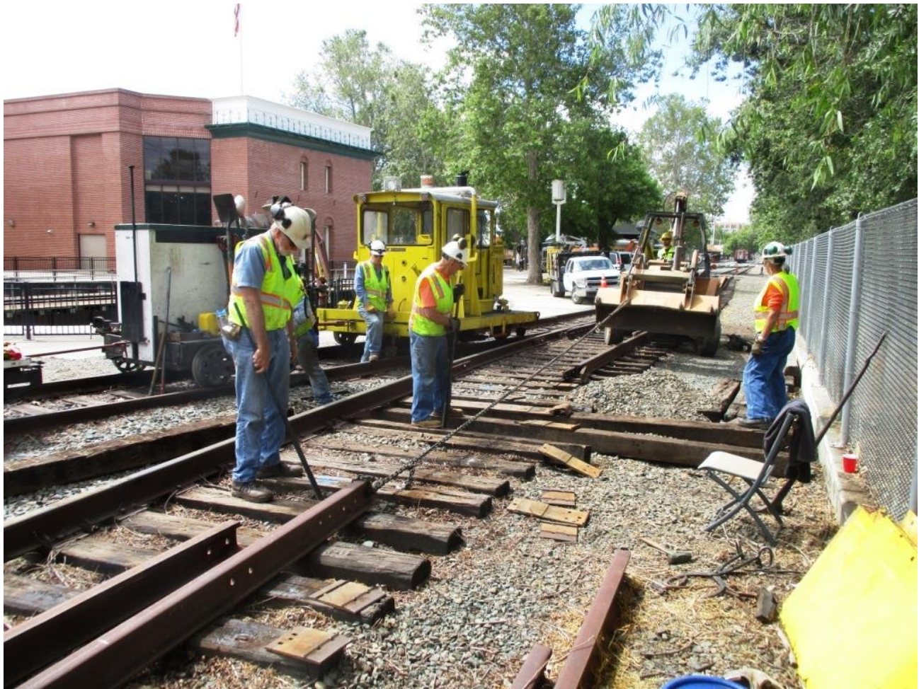
Chris on the back-hoe pulls the new rail down to where it needs to go
