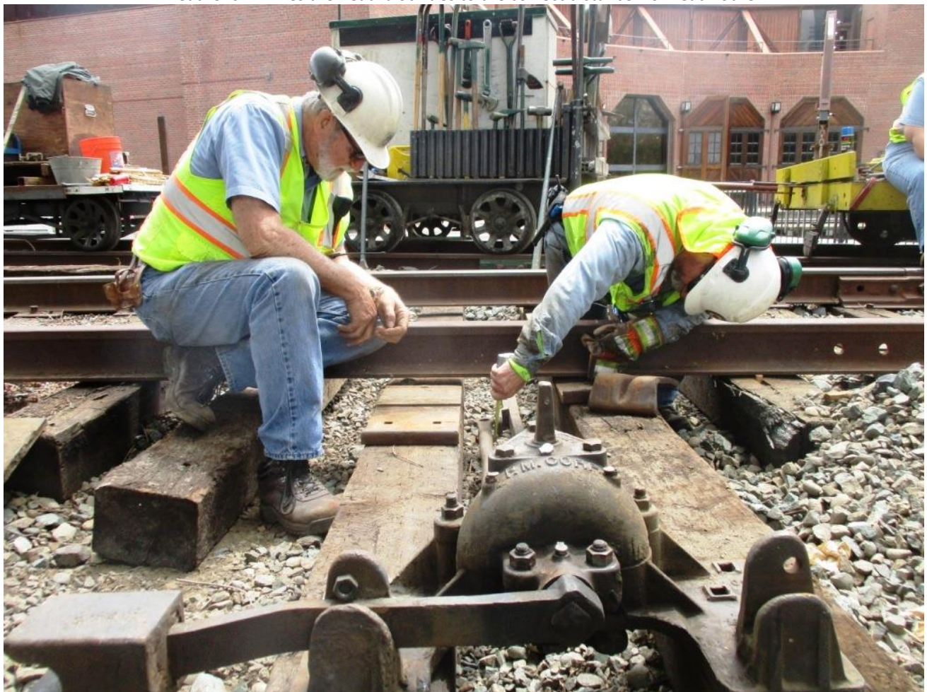
Alan and Joe take precise measurements for hooking the switch rod from the machine to the connecting rod between the rails
