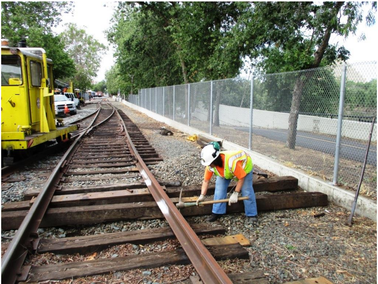
Pam digs a new tie-crib for the next switch-tie to be installed
